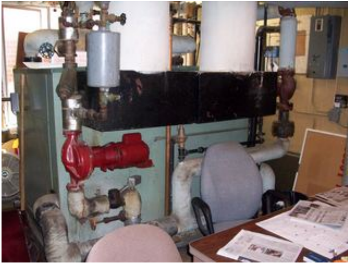
Gas Fired Hot Water Boiler
