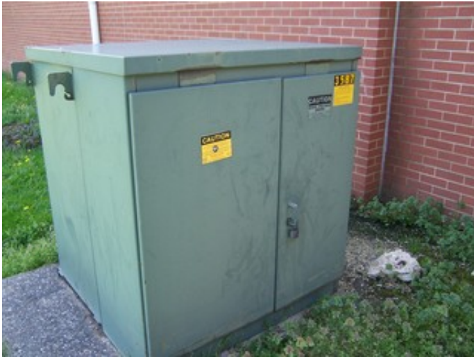
Pad Mounted Transformer
