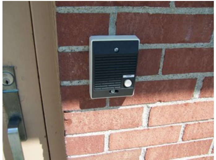
Exterior Buzzer & Intercom
