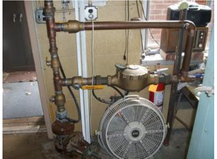
Domestic water piping
