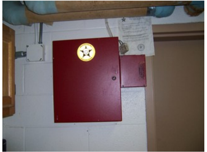
Fire Alarm Control Panel
