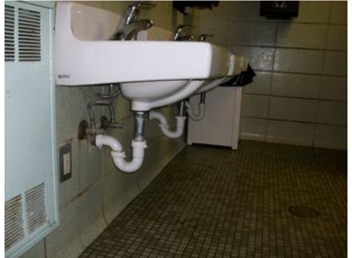
Sanitary drain below sink
