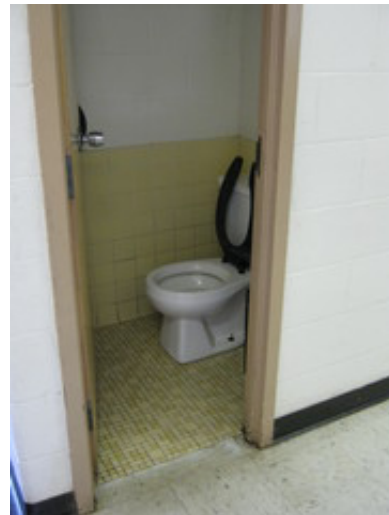
Non-compliant private toilet
