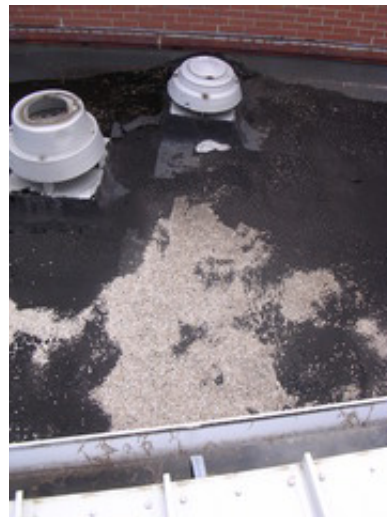
Typical built up roofing and flashings.
