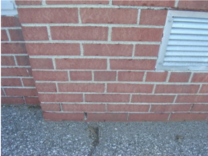
Typical foundation condition.
