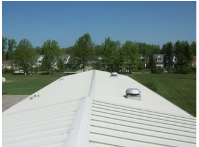
Roof top Ventilation Fans
