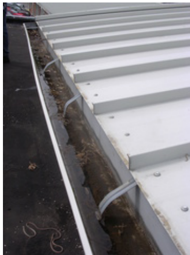
Typical standing seam metal roof and gutter condition.
