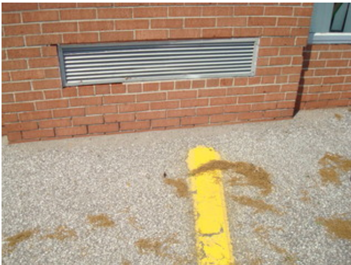
Tuck pointing needed at 1961 Original Construction
