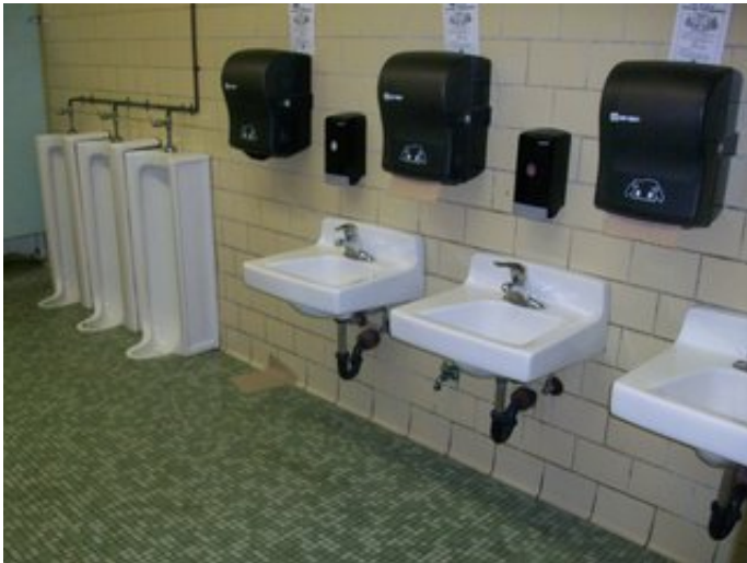
Toilet room fixtures
