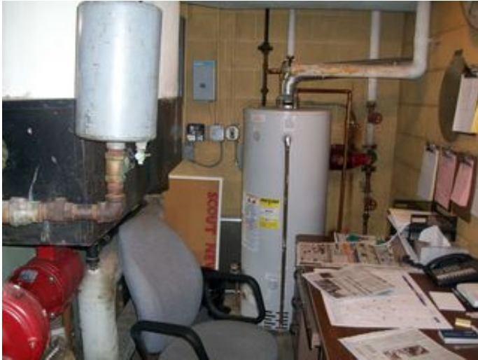
Domestic water heater
