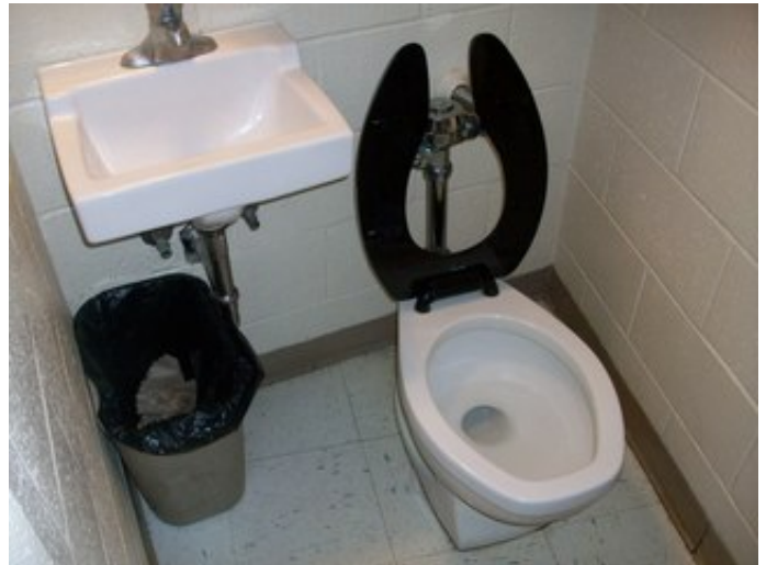
Toilet room fixtures
