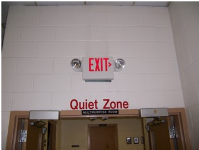
Wall Mounted Exit Sign
