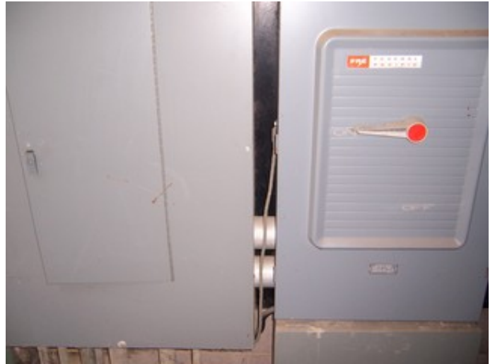
Main Electrical Switch & Panel
