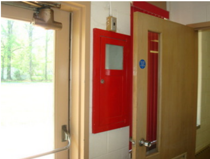
Fire extinguisher cabinet
