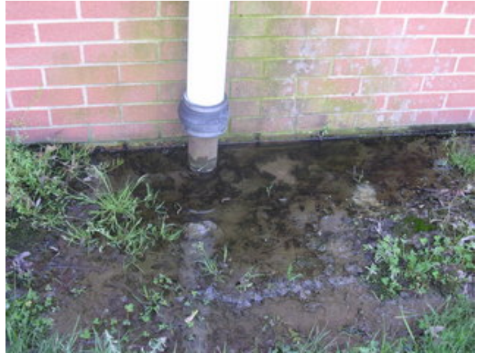
Condition at damaged underground drain tile.
