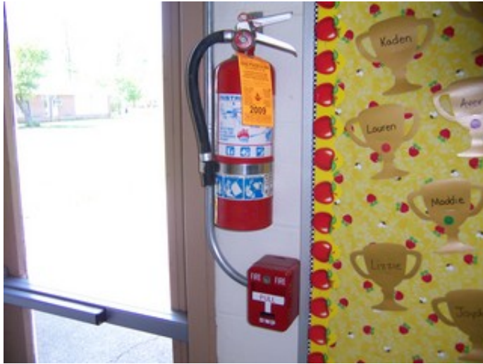
Fire Alarm & Device
