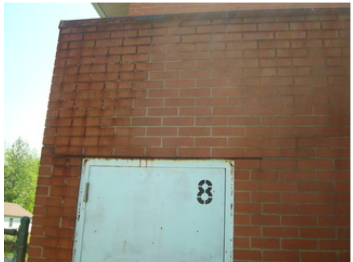
Lintel replacement needed at 1973 Addition electrical room
