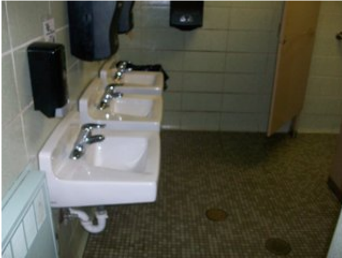
Sanitary drain below sink
